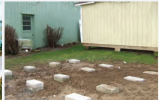
Concrete Block Site
